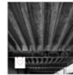
Rippenplatte Stahlbeton / L=8.97m, B=1.495m
