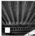
Rippenplatte Stahlbeton / L=5.99m, B=1.495m
