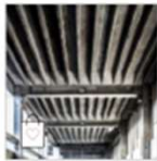
Rippenplatte Stahlbeton / L=5.79m, B=1.495m
