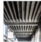
Rippenplatte Stahlbeton / L=6.84m, B=1.495m
